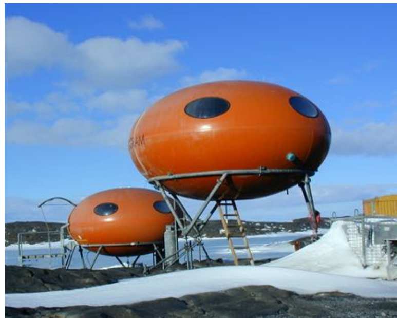
Fig 2, above. Field station on Bechervaise Island. "Googie huts", Tasmanian designed and built. Their 360° aerofoil structure keeps them free of snow.
